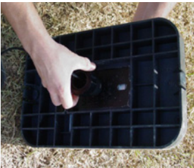
Figure 11 Feeding Antenna Cable
