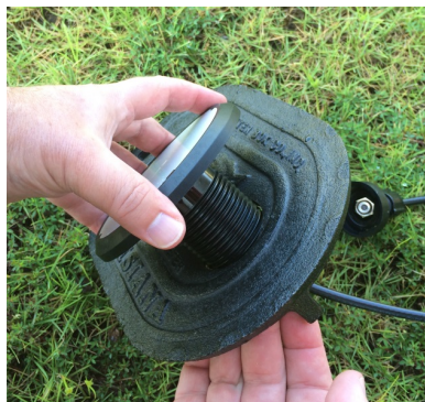
Figure 28 – Inserting the Antenna into the Pit Lid
