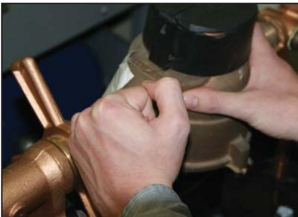
*Install water meter (manually)*
