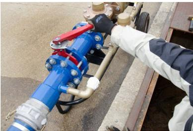
Figure 11 Back-Flushing the Meter
