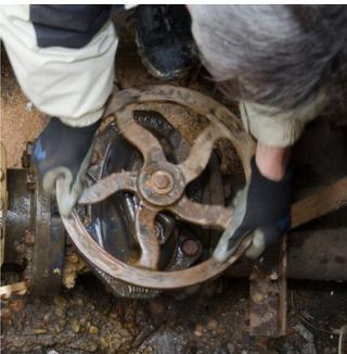
Figure 16 Isolation Valve - Downstream of the Meter Under Test
