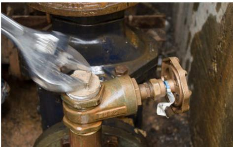
Figure 4 Remove Test Plug
