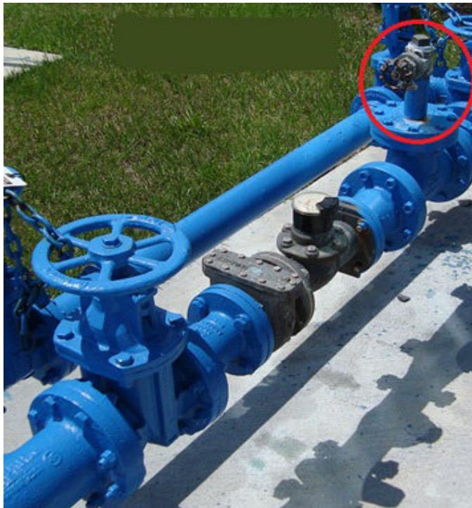
**Figure 2 HP Turbine with Test Tee Installed**
