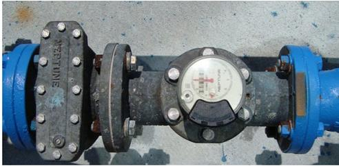
Figure 8 Register on Meter Under Test
