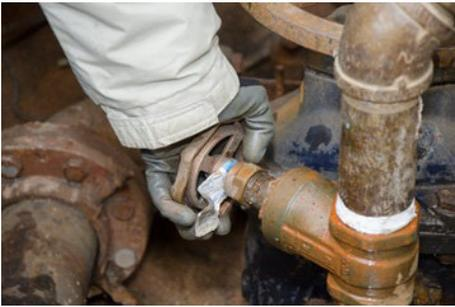
Figure 14 Test Riser Valve Attached to Meter Under Test
