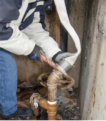
**Figure 5 Connect Fire Hose to Meter Under Test**
