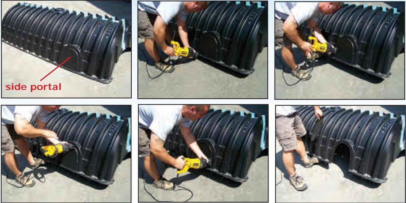
Following the guides on the side portal, use a reciprocating saw to trim out the opening to accommodate the HVLV Feed Connector.
